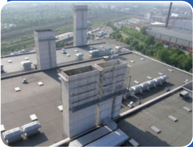
Exterior views of both exhaust air chimneys to be retrofitted
