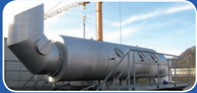
Volume resonator with cleaning facility
