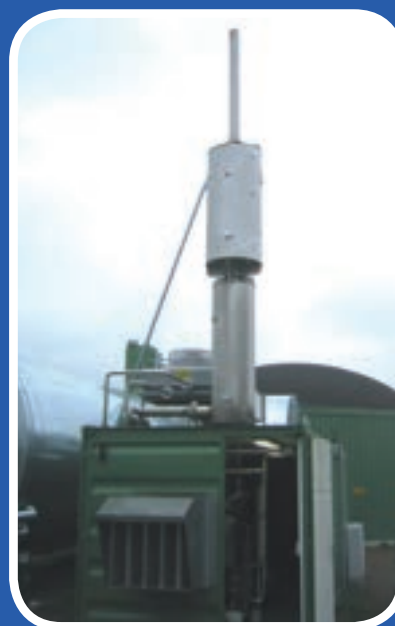
Housing for a biogas generator in a container with adequate silencer system
