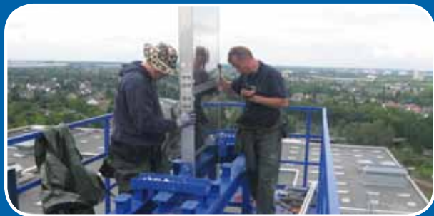
Installation of the 17.5 metre sections of plate absorber in the duct
